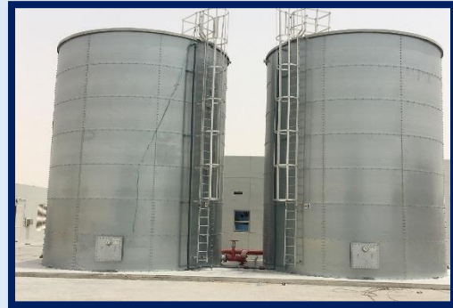
INNOVA TANKS CLEANING, DIC
