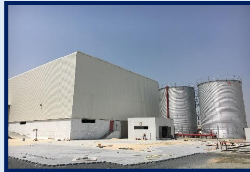
WAREHOUSE, G+M OFFICE FOR M/S VERSATILE FREIGHT SYSTEMS LLC, JAFZA, DUBAI
