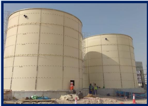
SUBSTATIONS FOR 1177MWP SOLAR PV PROJECT, SWEIHAN, ABU DHABI
