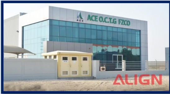
FABRICATION & STORAGE FACILITY FOR ACE O.C.T.G FZCO. JAFZA. DUBAI
